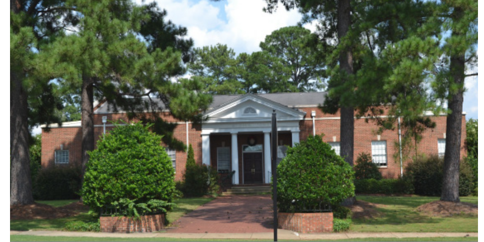
THETA TAU RENOVATION
