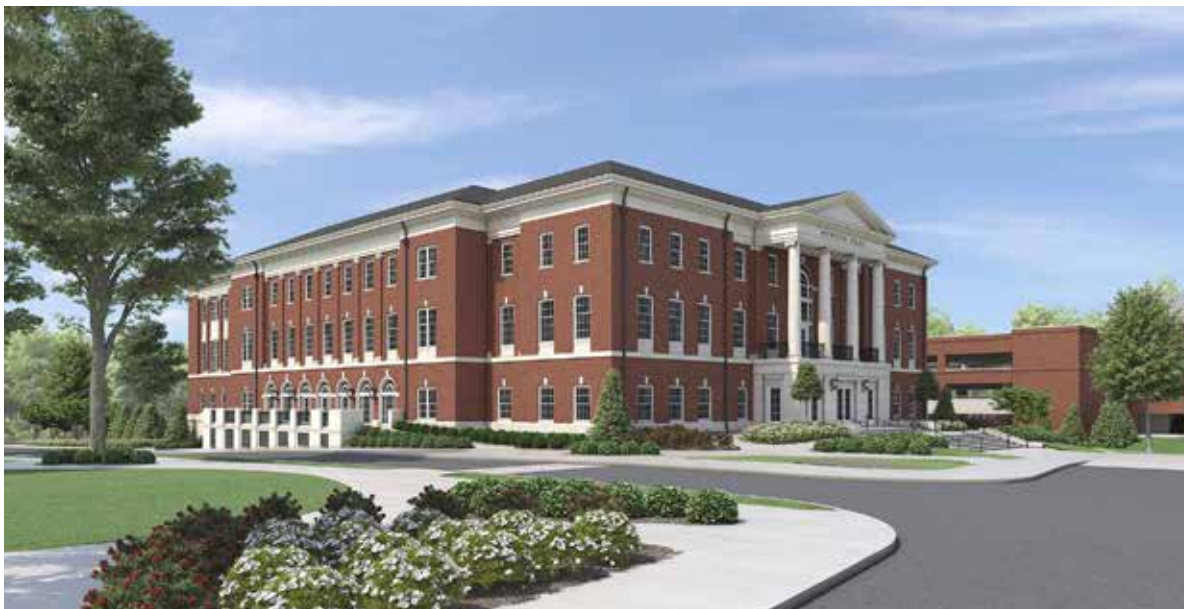
View from Stadium Drive
