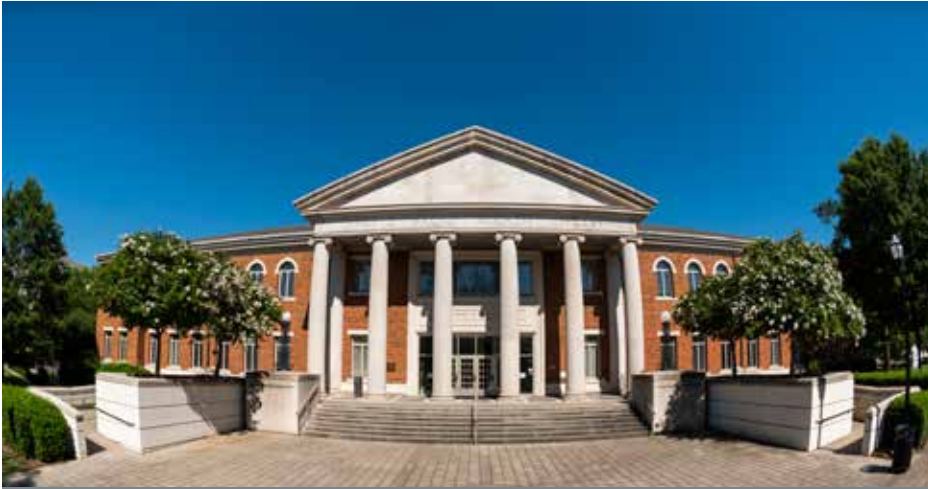
BRUNO BUSINESS LIBRARY RENOVATION
