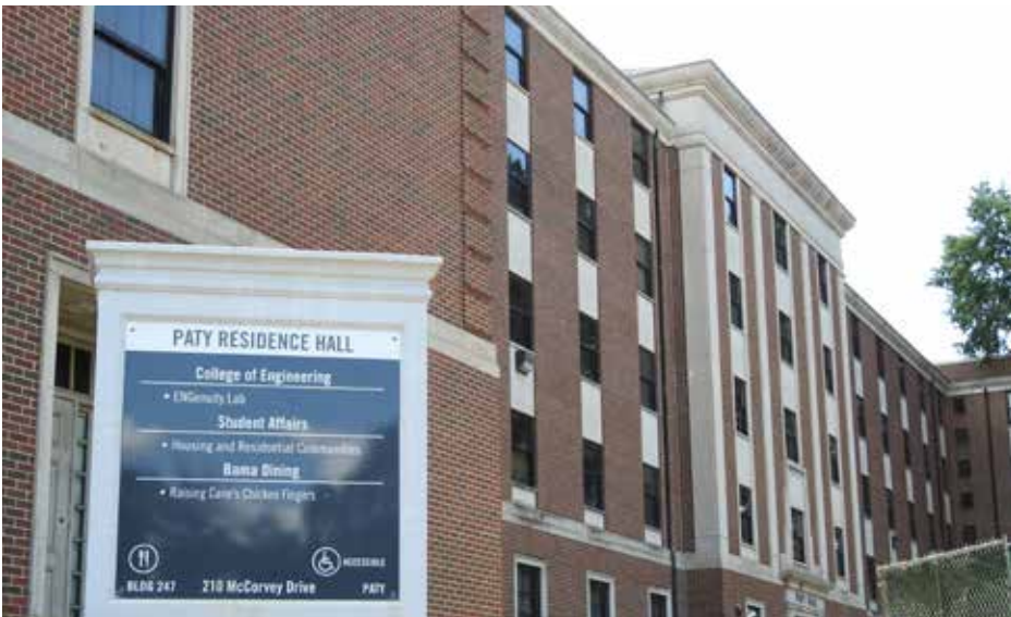
PATY HALL RENOVATION
