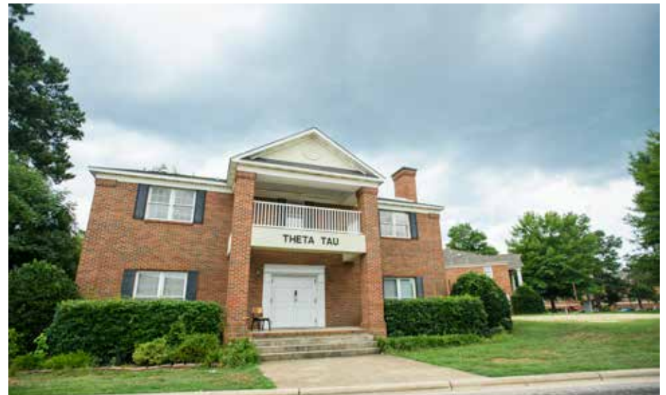
THETA TAU RENOVATION
